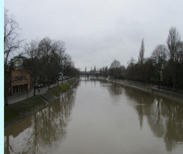
At York, the River Ouse has been lined and straightened. Photo © Robert Gamesby.
