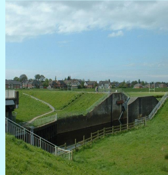
Spillway on River Wyre at Garstang, Lancashire. Photo © David Medcalf.
