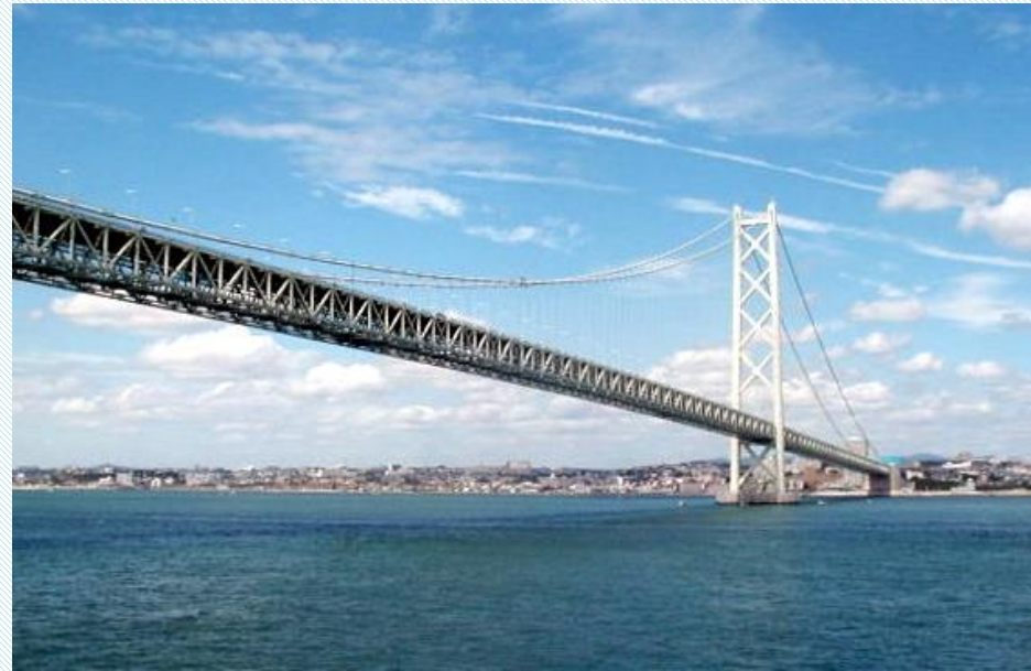
Akashi Kaikyo Bridge, Japan 1991m
