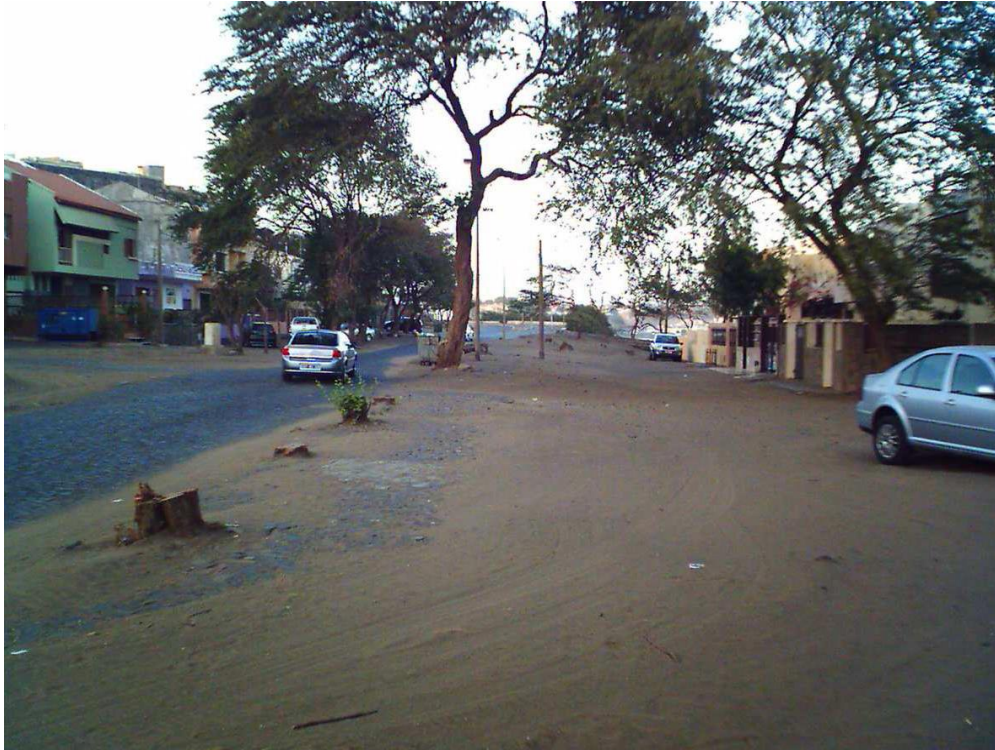
Fig. 2: Sand covering part of a main road in Praia, Cape Verde
